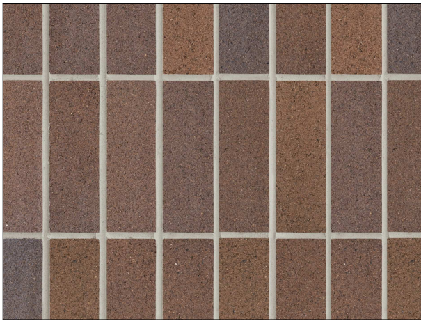
BWK(1) Face Brickwork Type 1 Bowral Blends - Bargo (10% Bowral Brown & 90% Gertrudis Brown) or similar
